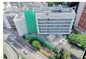
Commencement of Phase II of the School Enhancement Project.
